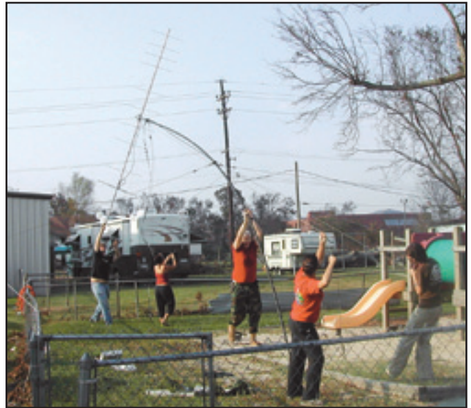
A team of Katrina volunteers from Rhode Island installs a temporary antenna.
