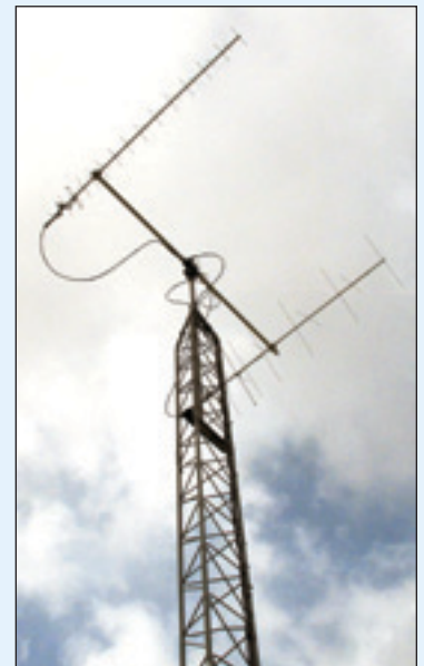
The satellite antenna tower at the Johnson Space Center Amateur Radio Club, W5RRR. It is equipped with M 2 circular polarized satellite antennas.
